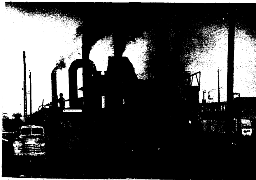
Figure 3. Continuous Plant during Operation.
